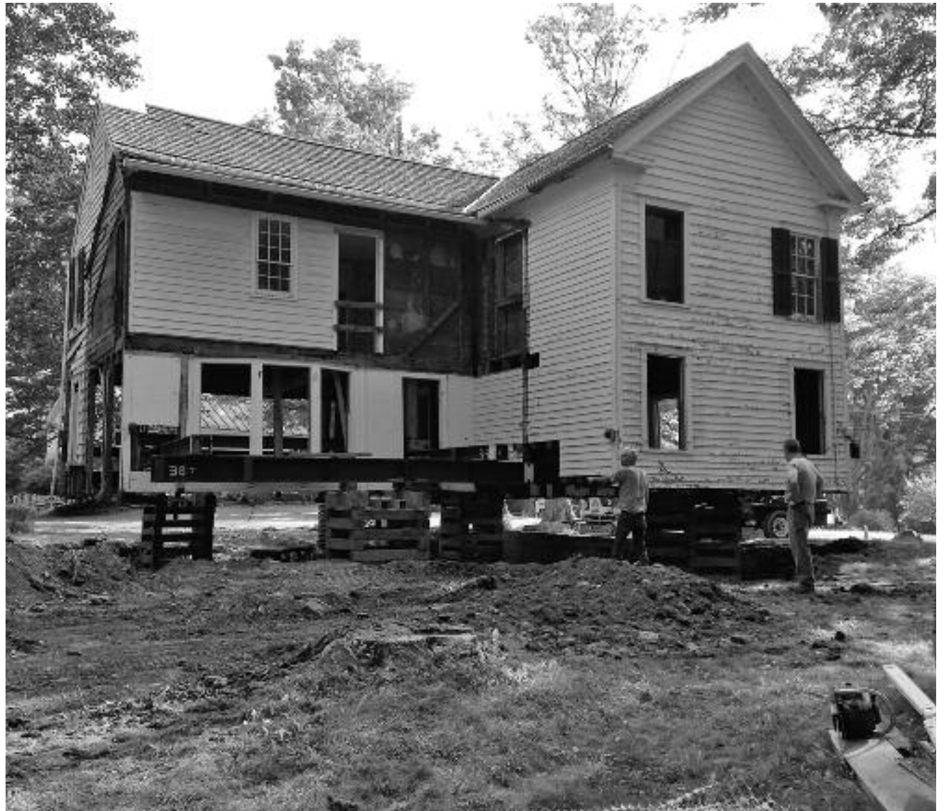
As part of the massive undertaking, Vazac had the foundation raised 36 inches and a fully insulated basement was dug, replacing portions that were just dirt.
